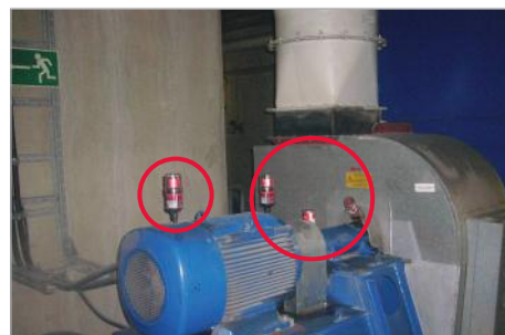
Lubrication of electric motor and shaft on a secondary air fan.
