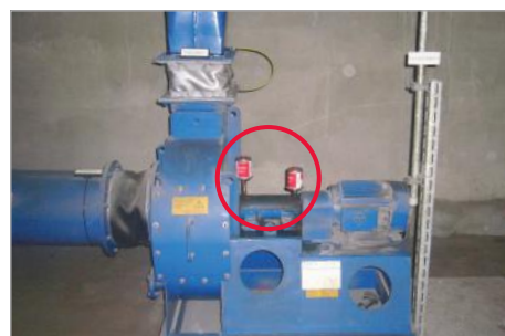
Lubrication of drive shaft on a fan
